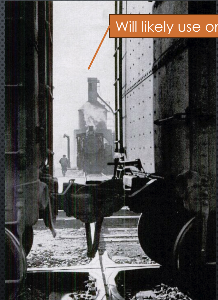
Cooling Tower on C&WC
